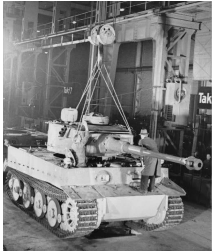
Nearly complete (note transport type tracks).
