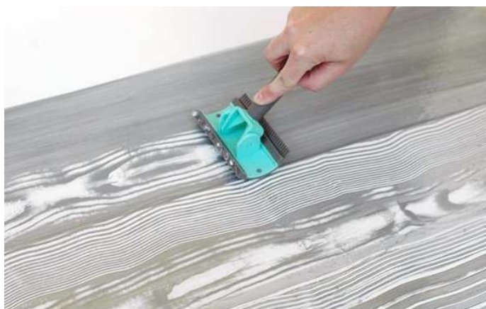
Real-world woodgraining with a rocker. Note the arched and curved grains that provide a natural look.
